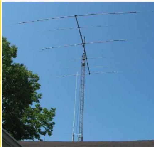
self-supporting crank-up tilt-over tower that seems to be about 40 feet tall. The tower itself seems to be structurally sound with some surface rust, but the steel cabling is rusted and broken. If nobody wants the tower, she is willing to pay to have it removed. Can anyone recommend a professional outfit that could do this for her?
